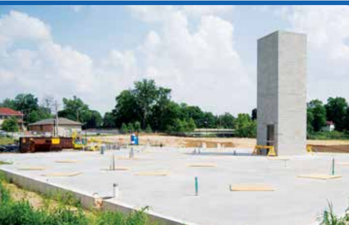
Mishawaka Campus construction
